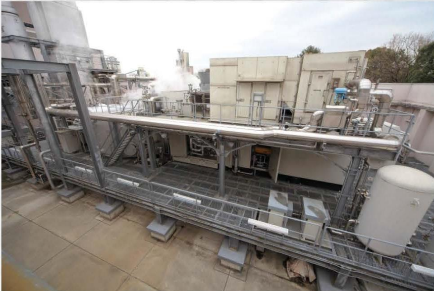
Waste Heat Boiler :WHB
