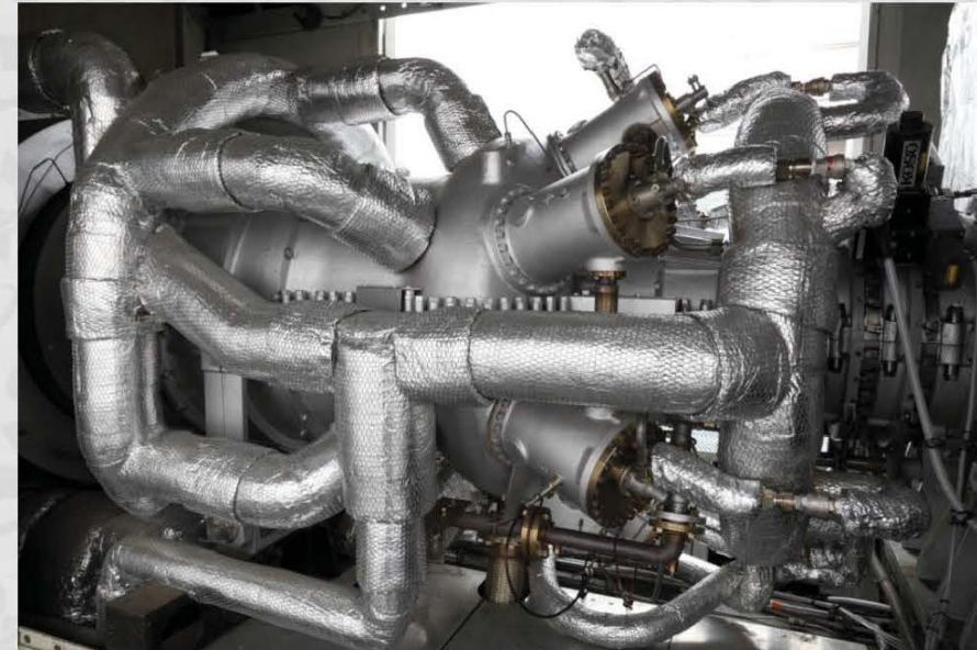
Gas Turbine Generator : GTG
