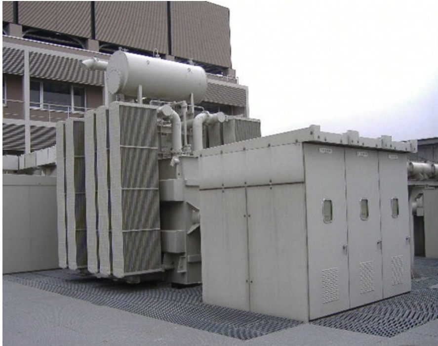
Fig. 4 RIBF substation. The front is a 66-kV gas-insulated substation with a VCB. The back row shows a transformer with a capacity of 25/30 MVA and the 6.6-kV metal-clad switch gears behind.
