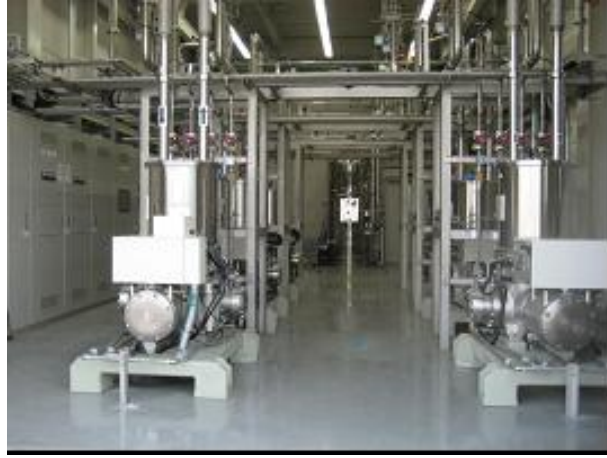
Figure 3 photos of the high-temperature superconducting cable cooling system
